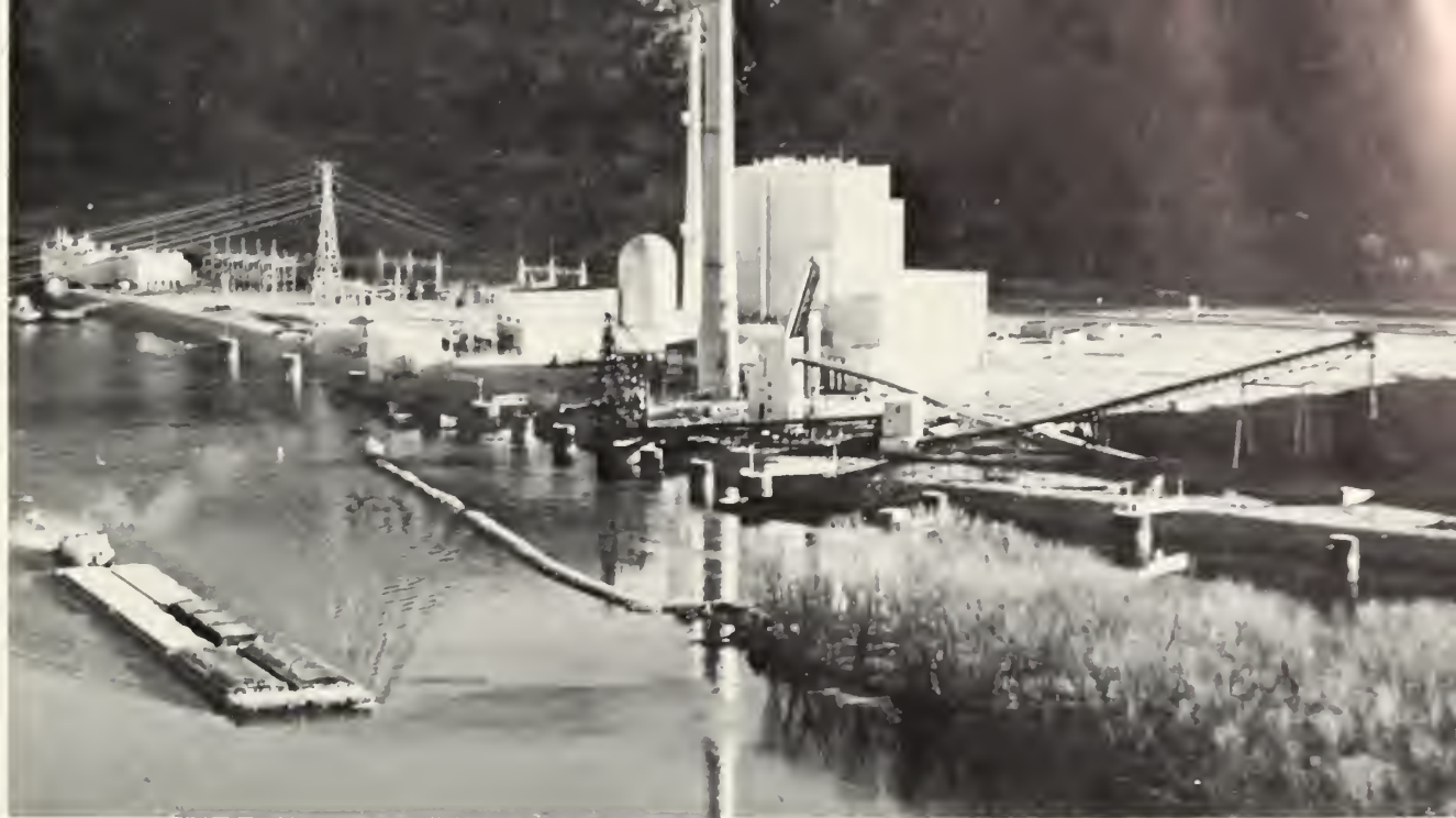
A 14,000 kW generating plant built in 1941, far left, contrasts with a 300,000 kW unit, center. An experimental 50,000 kW nuclear plant (round dome) was completed in 1969.
